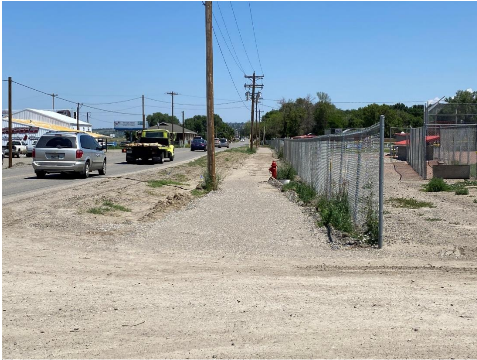
PHOTO 4: SIDEWALK CORRIDOR IN FRONT OF LOCKWOOD BASEBALL COMPLEX PREPPED FOR CONCRETE. RELOCATED WATER SERVICE METER PIT.
