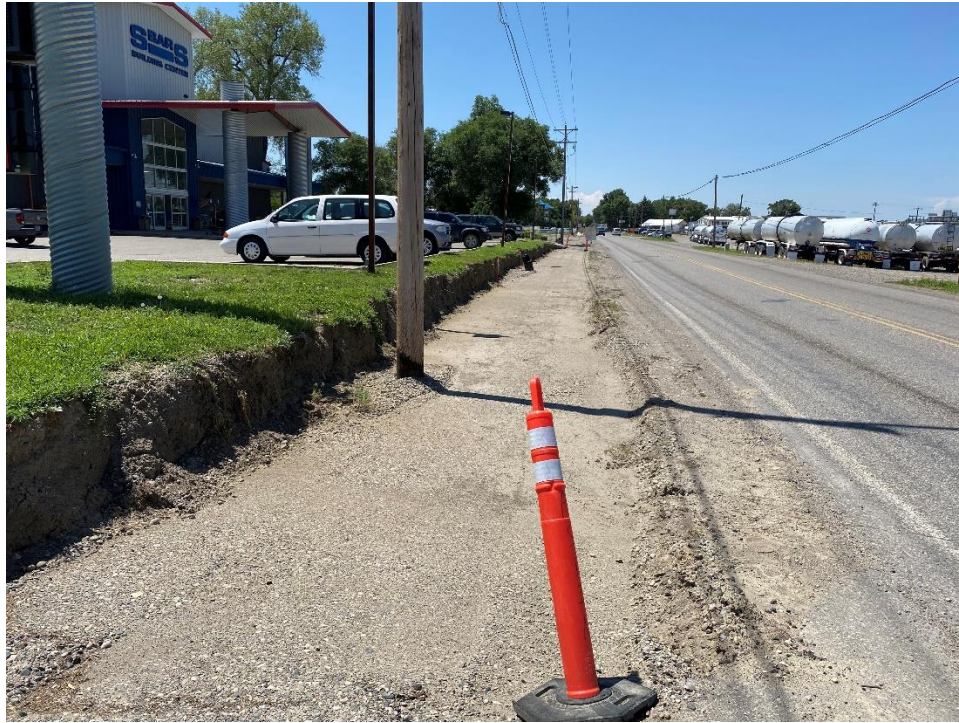
PHOTO 2: SIDEWALK CORRIDOR IN FRONT OF S-BAR-S PREPPED FOR CONCRETE AND RETAINING WALL CONSTRUCTION.
