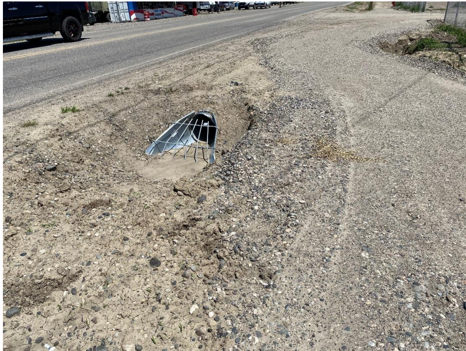
PHOTO 3: CULVERT EXTENSION WITH TRASH GUARD INSTALLED NEAR WEST APPROACH OF LOCKWOOD BASEBALL COMPLEX.
