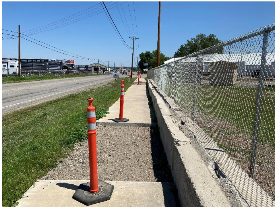
PHOTO 1: ANNEXED SIDEWALK WITH DAMAGED PANELS DEMOLISHED AND SLATED FOR REPLACEMENT. RELOCATED CHAIN-LINK FENCE.
